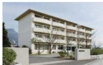
KU dormitory (Yashima area)
