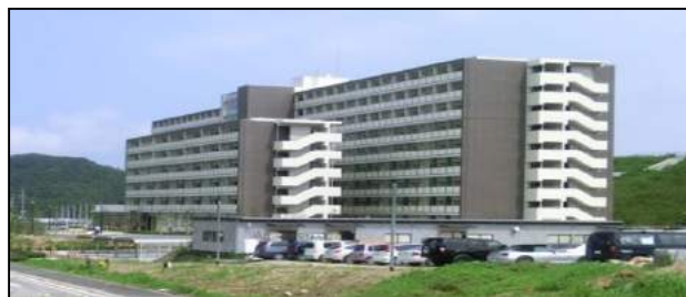
< Ito Harmony House – a dormitory for Japanese and International Students at Ito Campus >
