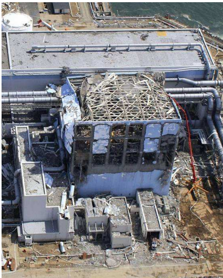
Air Photo Service Inc (Myoko, Niigata Japan)
